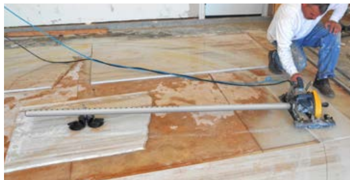
Cut circular floor inlays as well as curved countertops.
