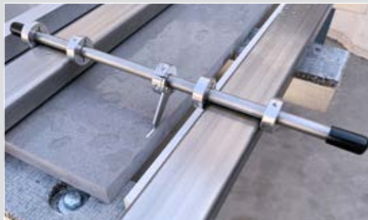
2. Place the tracks on cut line.
